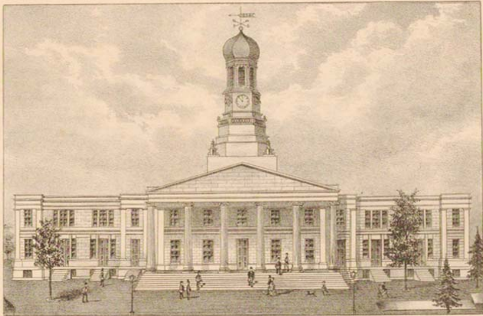
COURT HOUSE, NORRISTOWN, MONTGOMERY CO., PA.
